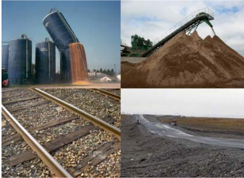
Figure 1.2: Some examples where the need to model granular materials is necessary (in clockwise direction) : Collapse of silo used for storing granular materials, Transportation of sand using conveyer belt, Granular ratcheting due to deformation in supportive granular rail bed in railway tracks, and on road networks, taken from [2].
